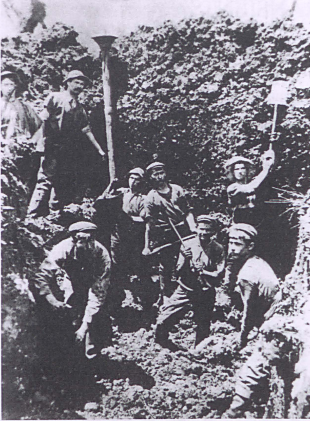
An example of deep potholing by a cooperative group with a hand pump at the back to dewater the hole. Courtesy of the Kauri Museum, A1.1992.915.71
