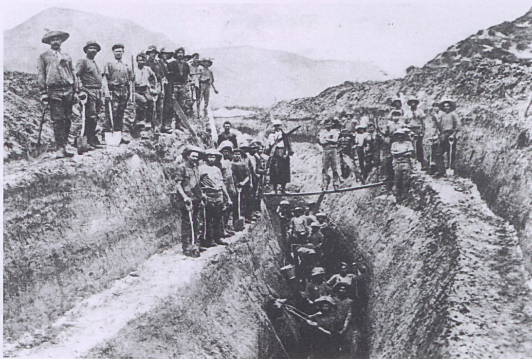
The Omamari Drain, one of many drains to allow digging in swamps as other gumfields became exhausted. (Despite the size of this undertaking it was not a financial success, see Jelich , p. 59) Courtesy of the Kauri Museum, A1.1992.915.78
