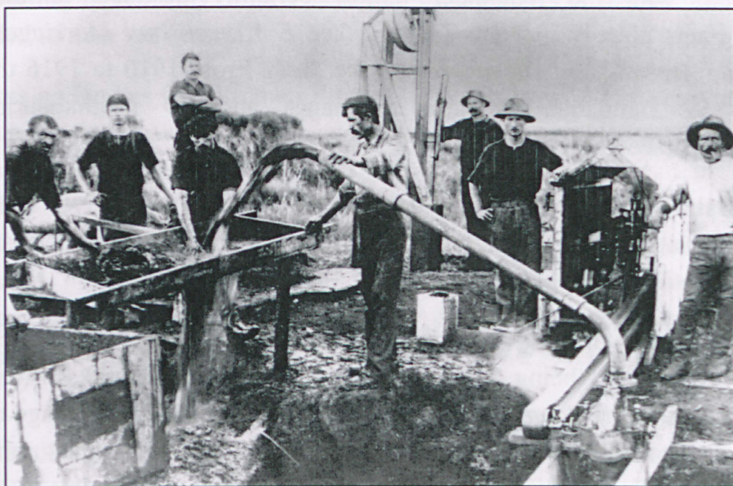
An early (c.1912) gum-washing operation using a motor-driven water pump to clean gum by washing over a metal screen. Photo courtesy of the Kauri Museum, A1.1992.915.26
