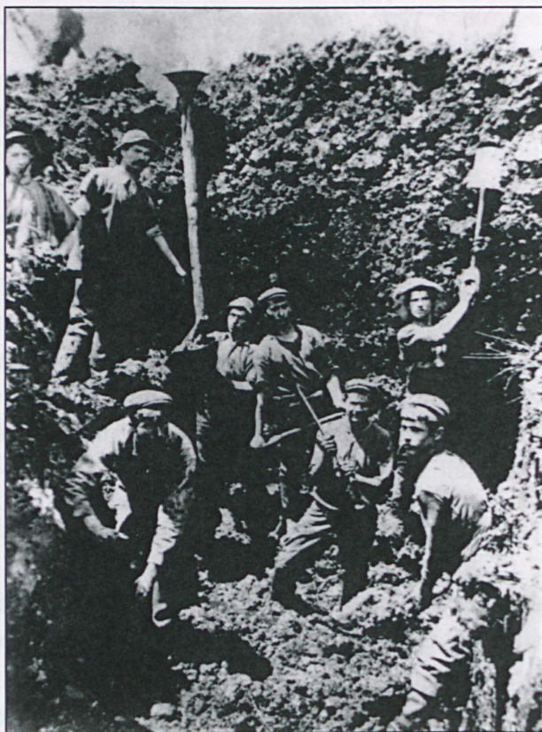
An example of deep potholing by a cooperative group with a hand pump at the back to dewater the hole. Courtesy of the Kauri Museum, 1.1992.915.71
